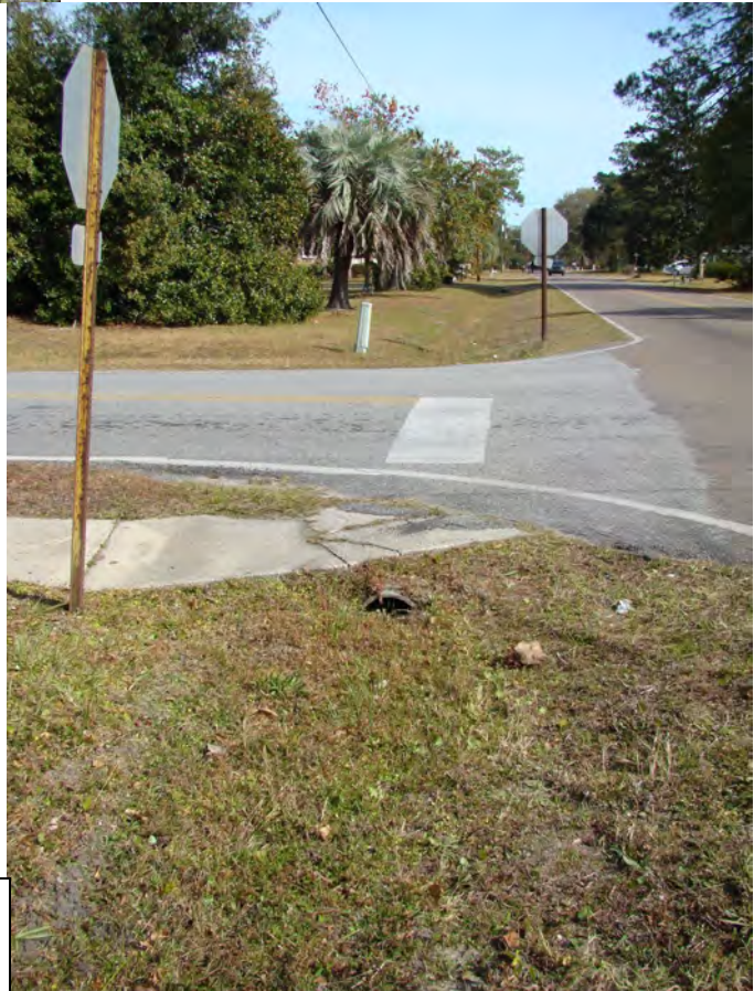
Photo 6 —Lack of sidewalk connectivity
